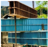
Pile Static Load Test
