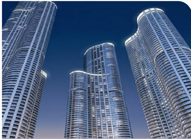
Lodha One World Project - Worli (Mumbai)
