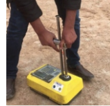
Field Dry Density Test
