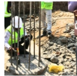
Pile Integrity Test
