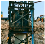
Pile Dynamic Test
