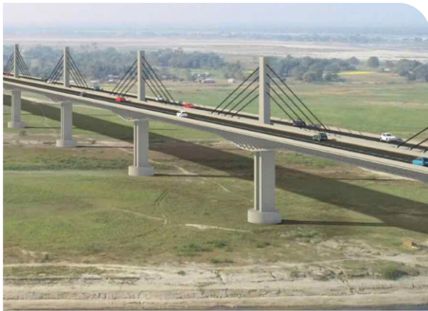
Dhubari to Phulbari Bridge - Assam
