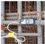
Mass Concrete Temperature Monitoring
