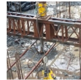
Pile Pullout Test
